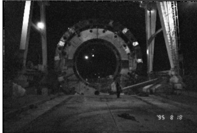
Figure 5. Assemble left cutter head shield and torque beam.
