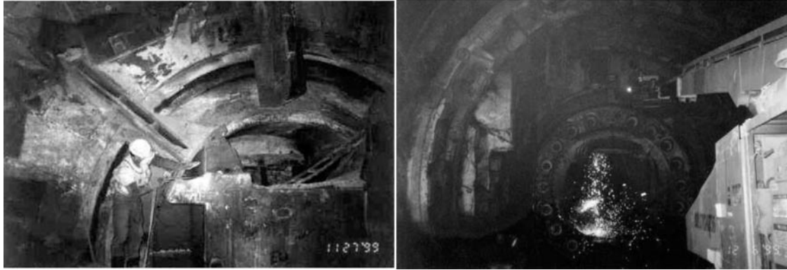
Figure 26. Dismantling of West Bound tunnel TBM by cutting.
