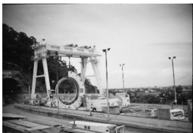
Figure 4. Assemble right cutter head shield and torque beam.
